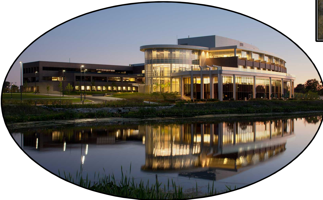
In-line Detention Basin at Delta Dental
