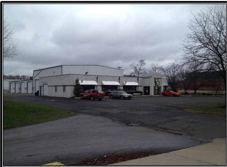
Jolly Rd Commercial Corridor Enclosed Pipe
